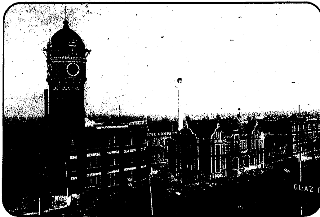
Clocktower under construction, 1907.
